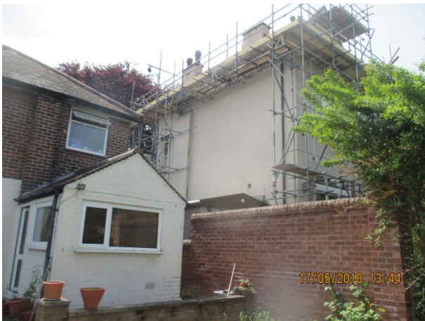
Looking west towards no. 3.
