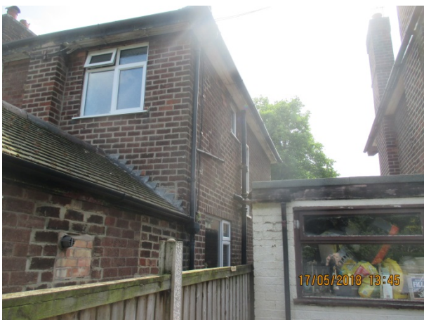
Looking south west towards boundary with no. 7.
