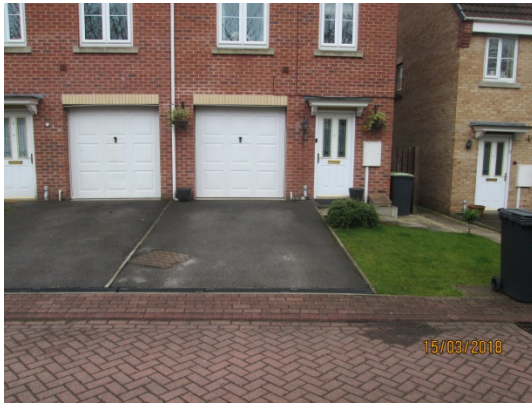
Frontage of garage and existing driveway.
